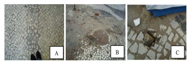
Fig. 5 A - Bad intervention, B - detachment and C - staining.
