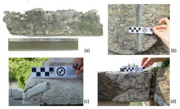
Fig. 2 (a) Lead plate; (b) Light staining on a gneiss block; (c) Lioz limestone area with restored part; (d) Substitute piece on a gnaisse block.
